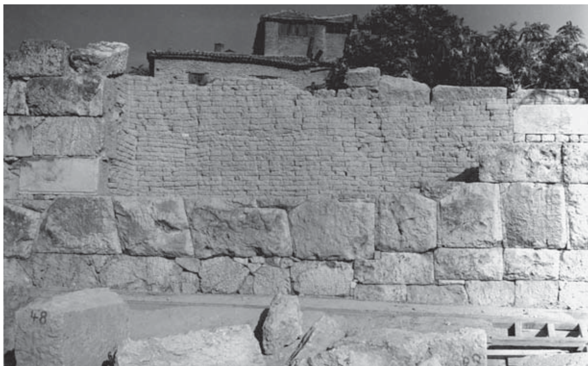
Fig. 2. Section of the Themistoklean Wall west of the Sacred Gate in the Kerameikos, with repairs by Konon and Demosthenes (Travlos 1971, 173, fig. 223) (DAI, Ker. 6006 [I]).
