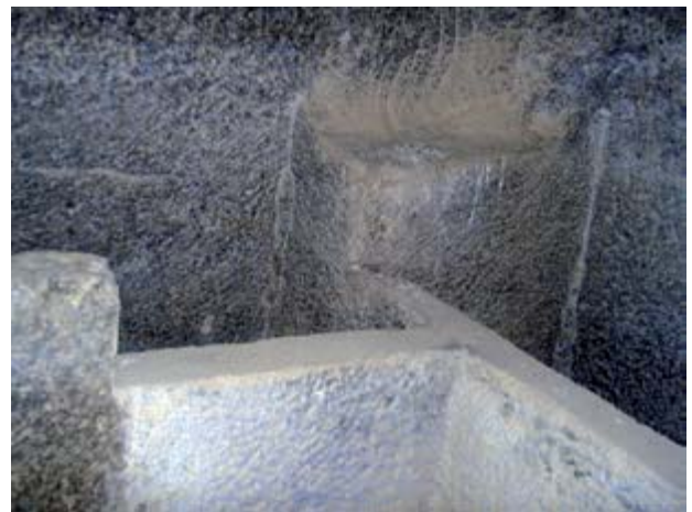
Fig. 11. CT3, left inner corner seen from the opening.
