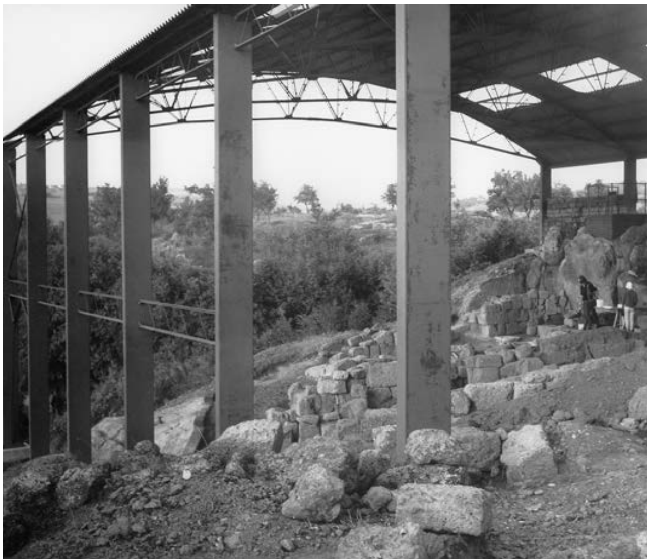
Fig. 30. The old Capannone 1965–2002. Photograph by B. Blomé.
