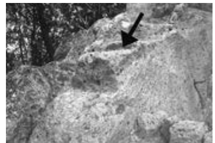
Fig. 16b. Close-up view of the fix measuring point for all levels, located at the level of 171.17 masl.
